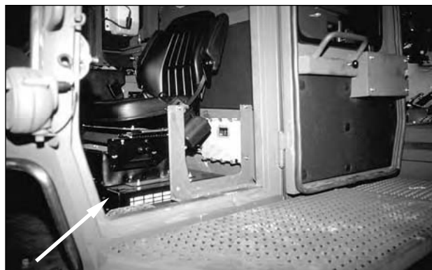
Air-Conditioning Unit, Under Operator's Seat.
